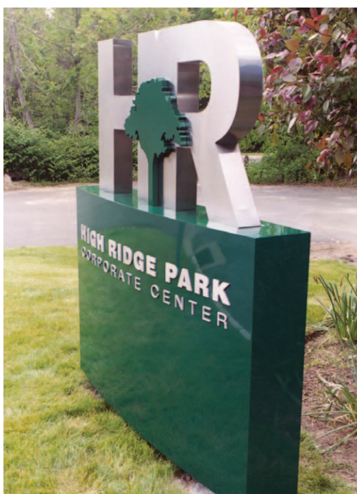
The 4-by-6-ft. base with painted aluminum composite panels over an all aluminum structure, with ¼-in. stainless steel flat-cut letters. The HR is 24-in. fabricated stainless steel letters; tree logo is ½-in. aluminum.
