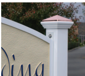
Copper cap finial on PVC post; 1/4-in. flat aluminum stock bonded to HDU sign for post mounting
