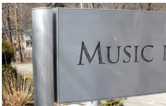
Illuminated lettering with perforated translucent film; sanded aluminum with clear coat
